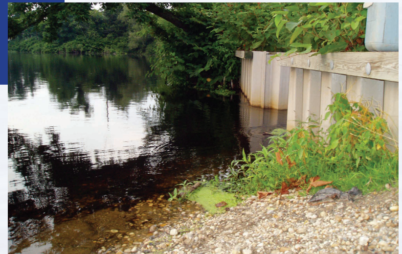
AREA AT UPPER MILLS SPILLWAY CLEARED OF LUDWIGIA
