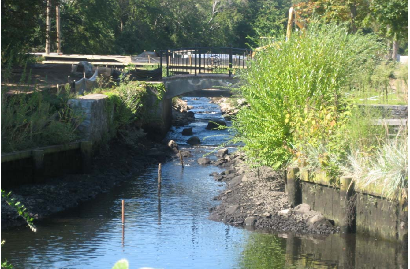
Grangebél Park Rock Ramp Fishway, Peconic River, Downtown Riverhead, NY. Installed February 2010.
